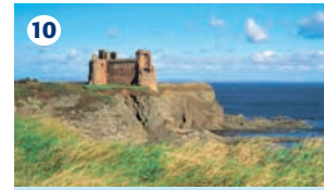
10 TANTALLON CASTLE – Set on the edge of the cliffs, the castle was a stronghold of the Douglas family. It features earthwork defences and a massive 50ft-high 14th century curtain wall with towers.
