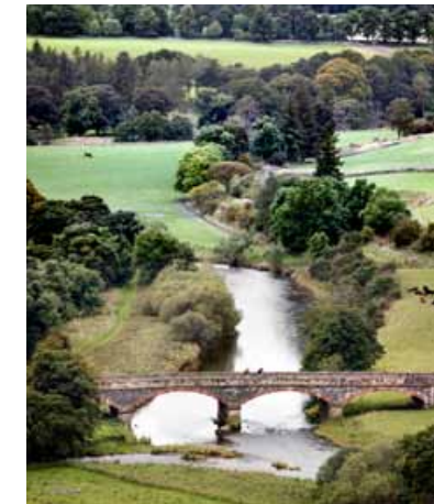
Mertoun Bridge from Clintmains
